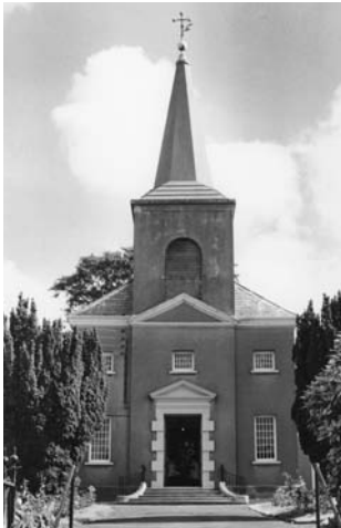
Fig 1: Knockbreda Parish Church of 1735, by Richard Cassels, photographed in 1980 (JSC).
