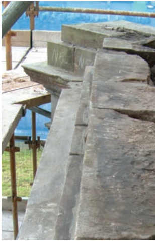
Stone cornice during work, Greg Mausoleum.
