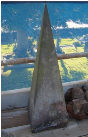
Work in progress, Rainey Mausoleum.
